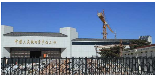
Museum facade under construction
