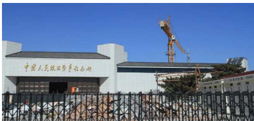
Museum facade under construction
